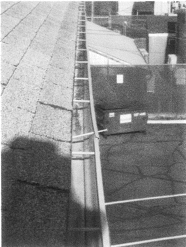
Photos 5 & 6 – shingles granules in gutter
