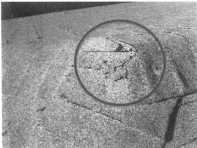
Photo 7, 8 & 9 – broken shingles
