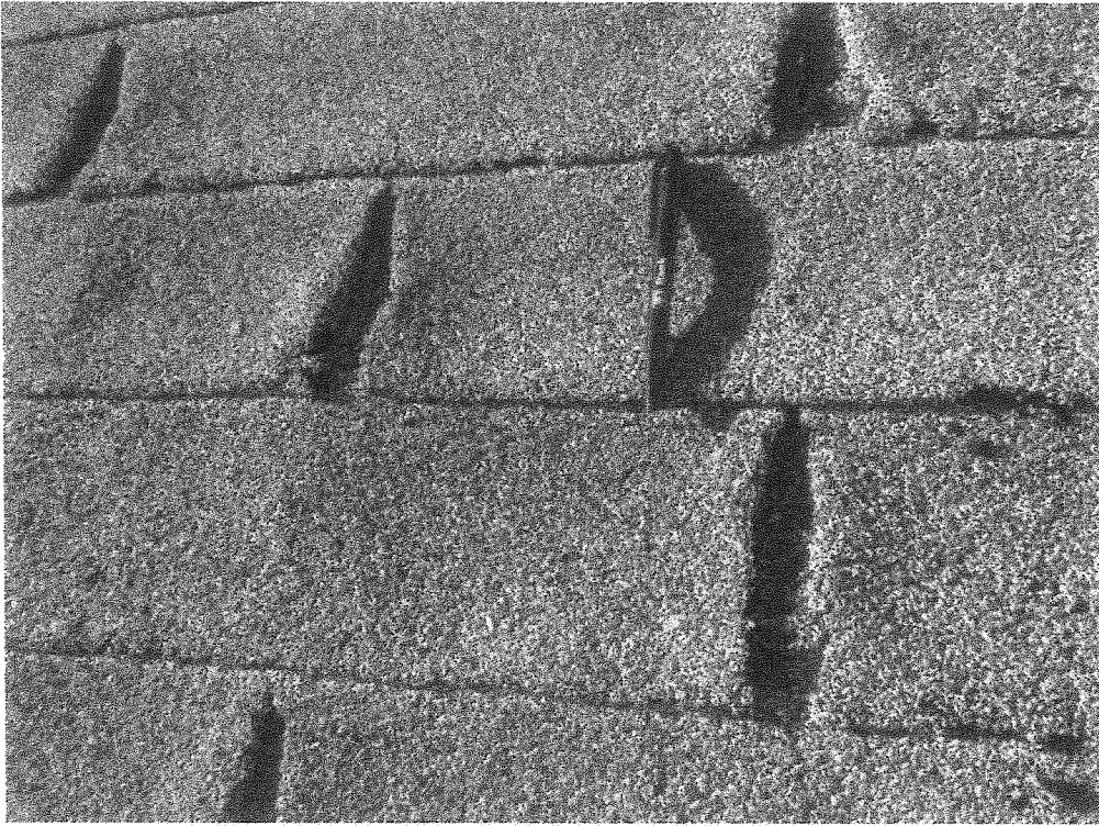
Photo 1 – curled shingles (note pen shadow line)
